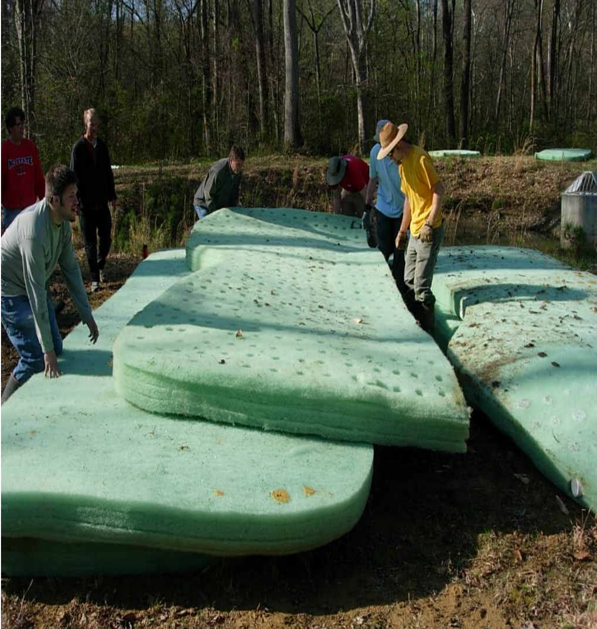
Large islands with pre-drilled holes move moveable by groups of 4 to 5 people.
