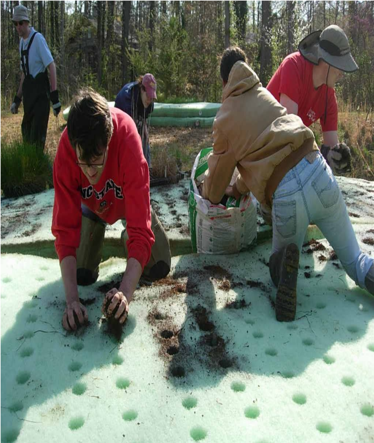
The holes were filled with peat moss to “jump start” plant growth.
