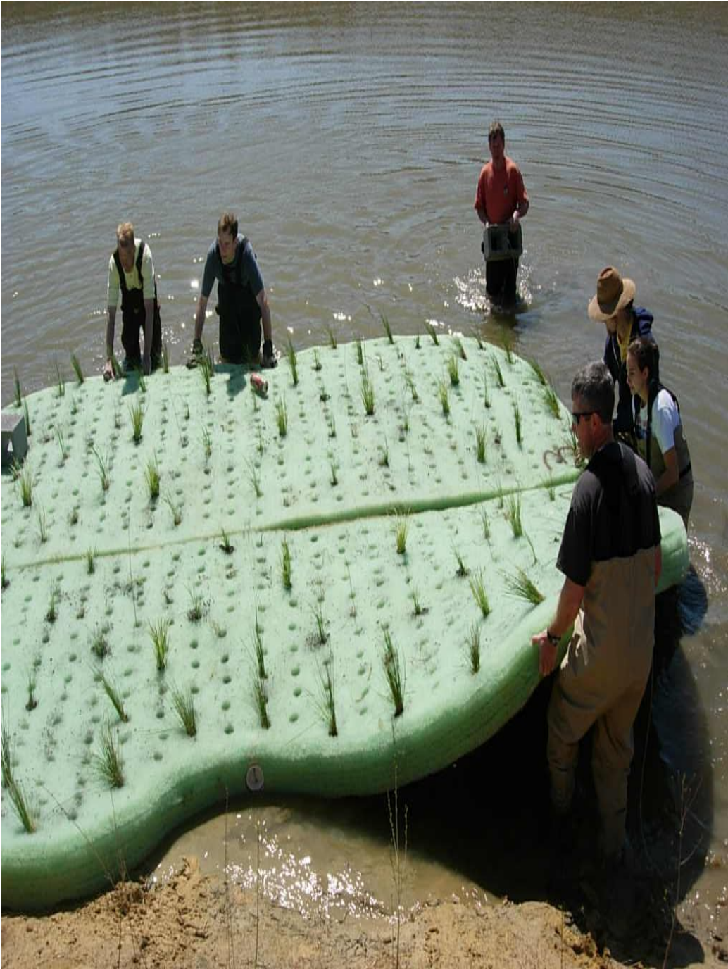
Floating the islands was relatively simple. They were anchored” using cinderblocks tethered to each corner of the island.
